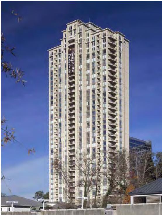
It looms over Atlanta's impressive skyline and ranks as one of its most impressive structures. But the gargantuan Paramount at Buckhead project is more than just one of Atlanta's largest and most impressive buildings. It is, in fact, one of the tallest and most impressive residential concrete tunnelform projects in the world.
