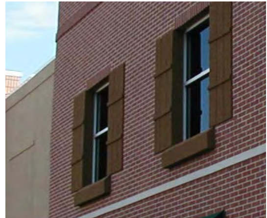
Using Dryvit Outsulation, windows were extruded out and the cuts and shapes were made to simulate window sills, shutters, and window boxes.
