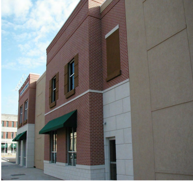
Two layers of Dryvit's intermediate mesh were used on the lower part of the building for added impact resistance in high traffic areas.
